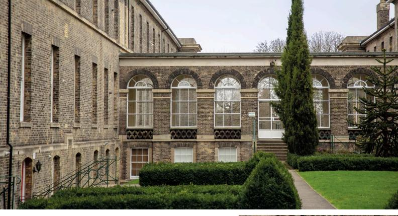
Our scope of works here comprised: roof repairs including slate repair and replacement and asphalt cleaning and painting; cleaning and flushing all rainwater goods; brickwork and render repairs; repairing, easing and adjusting all timber and metal casement windows and external doors, and replacing external floodlights.
