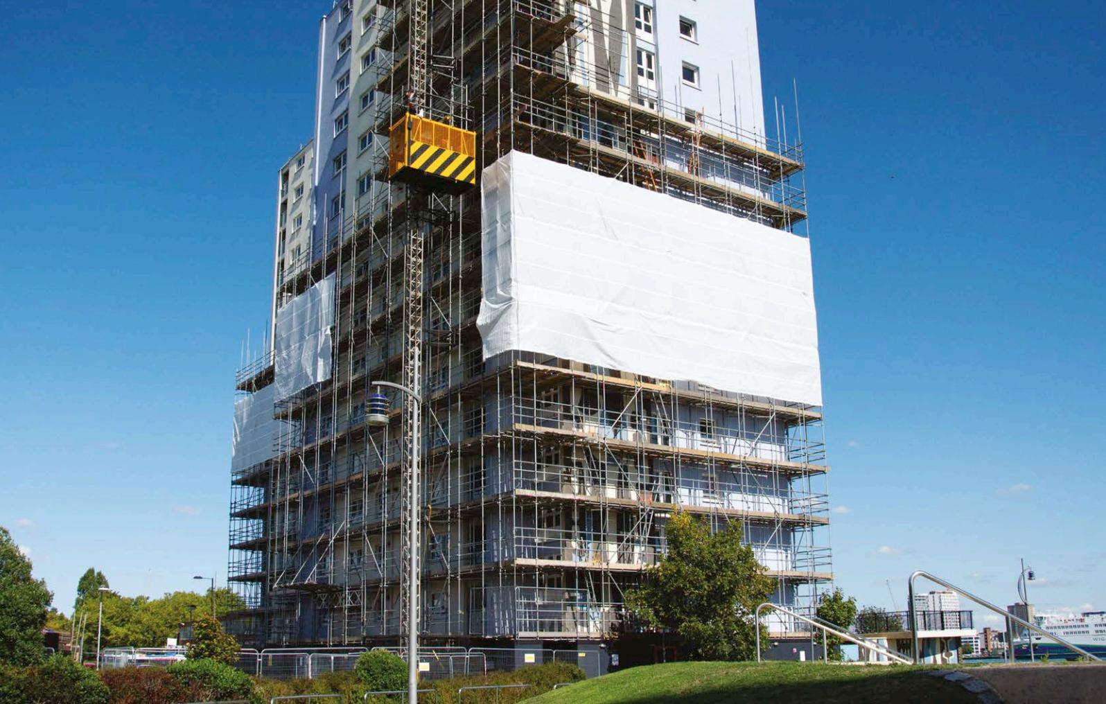
This required that Axis collaborate with Pellings and EWI manufacturers to review the original Employer's Requirement to establish an enhanced specification that exceeded the requirements of the current regulations and that was also practically deliverable on site: specifically, a replacement EWI system that met BR 135 classification (tested and certified to BS 8414).
