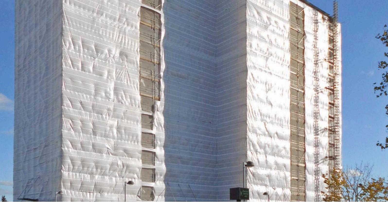
The works require that Axis erect designed scaffolding to enable access to all elevations of each block and fix a fire retardant Monarflex sheet to the scaffolding to protect the elevations from the harsh coastal and weather elements.
