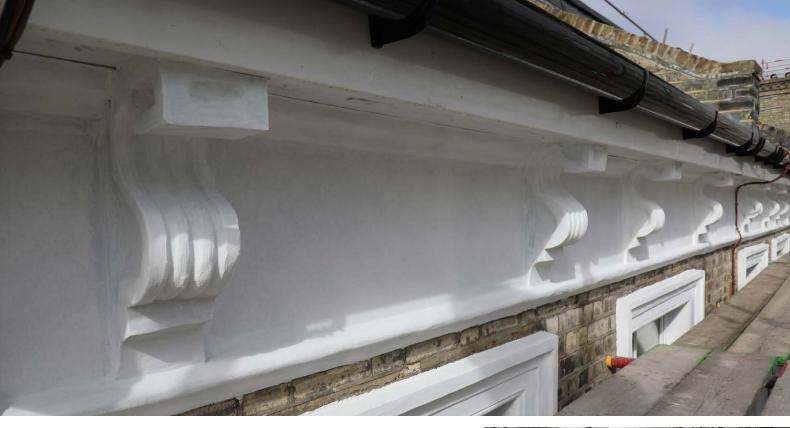
Some balconies were leaking, so we renewed all the asphalt to the balconies and drip edge details. In addition, we removed and renewed the asphalt steps. The team fully re-plastered and decorated all communal areas, with new carpets installed. We installed Aereco ventilation units into the flats, which are designed to manage moisture content.
