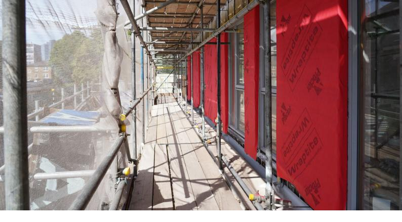
In addition, the team carried remediation works to resident balconies which involved the removal and replacement of the existing timber cladding and decking with non-combustible cladding and decking.
