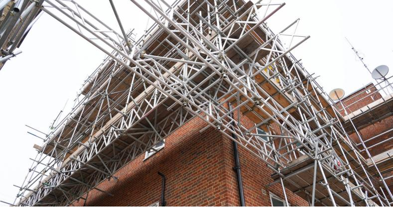
Our fully qualified Retrofit team installed External Wall Insulation to three blocks and replaced the roofs at two blocks, also extending the gable ends on one to protrude the insulation.
