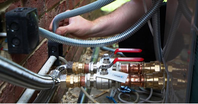
Our team re-sited the garden path to accommodate installing the ASHP outside the property; and despite the challenges of confined space under the stairs, we fitted the buffer vessel and most of the pipework here, upgrading the pipework to 35mm and 28mm.
