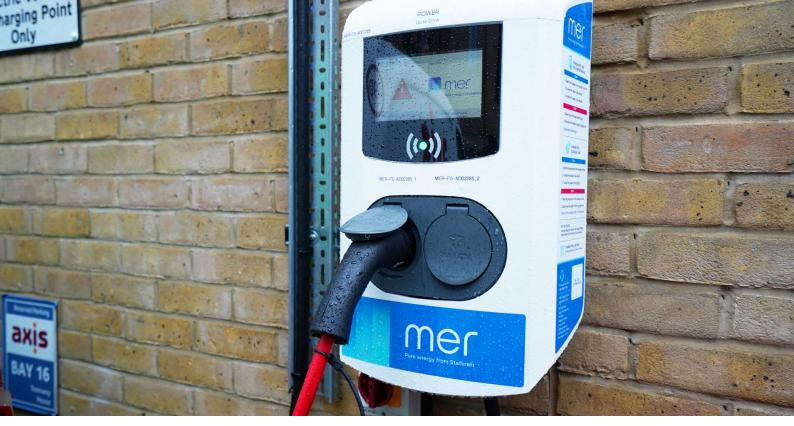
Each charge point offers remote monitoring and real-time usage date, allowing us to effectively manage our charging points and ensure they are ready for operation.
